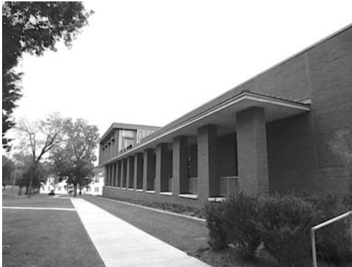
Fig 3 Thompson Center porch as shading device.
