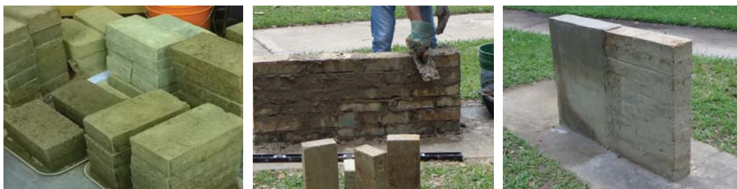
Figure 4: Earth block wall components and construction: earth blocks (right), wall during construction (center), and completed wall (right). Source: (Author)
