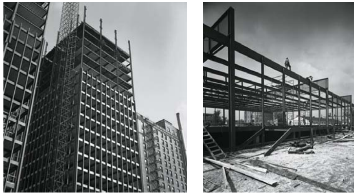
Apartment building at 860–880 Lake Shore Drive under construction. The photo shows the structural columns and the non-load-bearing I-beams.
