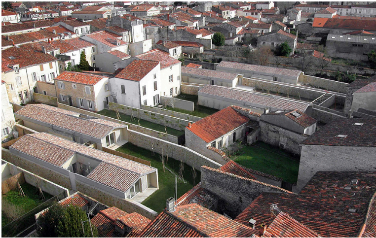
Figure 3: Ilot de l'Arc de Triomphe in Saintes: view from above of the general intervention (Source: BNR studio, 2021)
