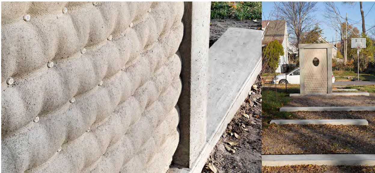
Figure 1: Detail and context view of Fabric Formed Poured Earth wall mockup installed permanently in Detroit. (Source: Rearick 2020)
