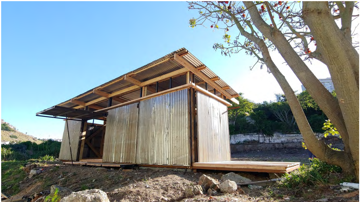
Figure 6: In realizing this work in South Africa, the designers worked as bricoleurs, developing a community makerspace using only common tools and reclaimed materials. The resulting project, which cost less than $1500, has successfully changed the manner in which new projects are developed within this community. (International Design Clinic, 2020)
