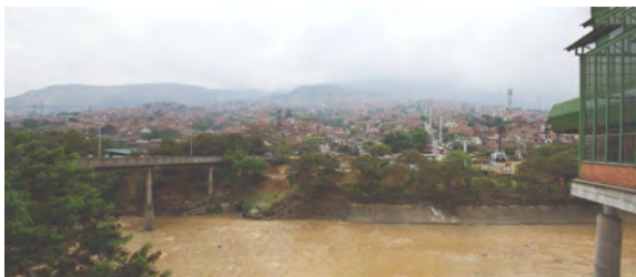
Figure 3: Medellín river canalization and the informal neighborhood of Santa Cruz (Author, 2018)
