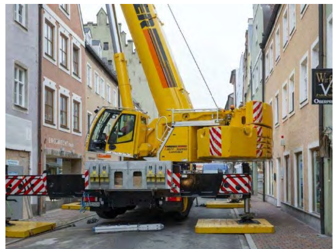
Figure 2: Crane set-up. (Dalhgruen 2012)
