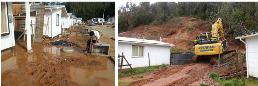
Figure 3: Images of Villa Horizonte under floods and landslides in 2013 because of lack of retaining walls and rainwater collection. Credits: Soychile.cl, Tomé al día, (2015).
