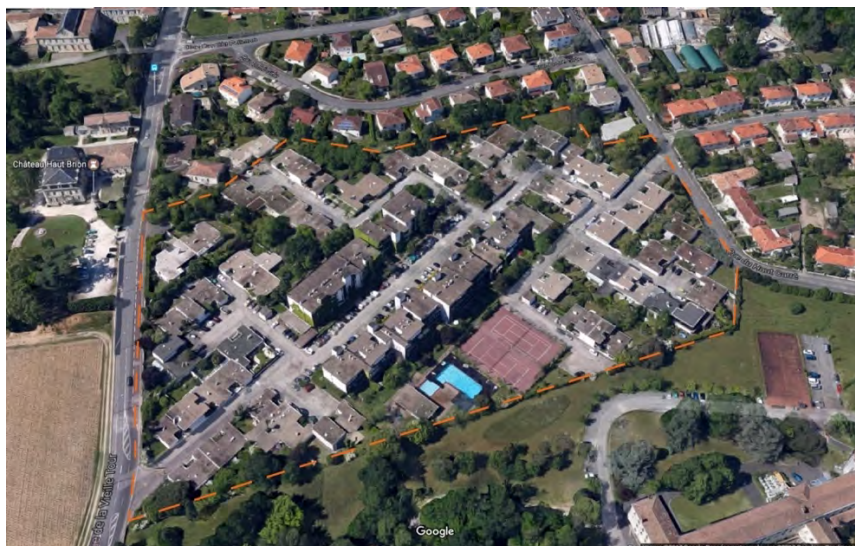
Figure 1: Hameau de Noailles, Talence, France; Salier, Courtois, Lajus and Sadirac, architects, 1968-1973. Aerial photo. Source: Google Earth 2020.
