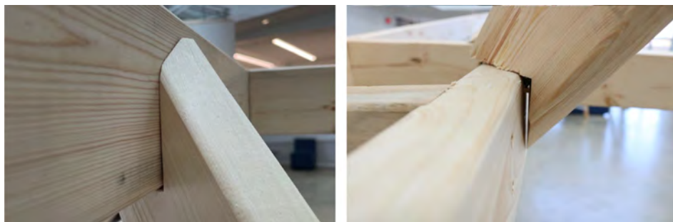
Fig. 9. Images highlight differences in tolerances incurred during the assembly process.
