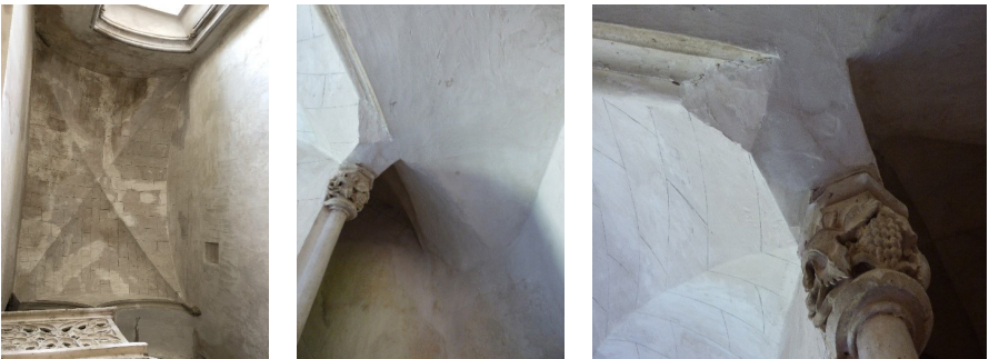
Figure 3. In the first image we see the problem in the outline of the stair space whose edges do not coincide at the vertices. The second and third images show problems of joints and geometry posed by the incorporated mullion, originally the top or square post of the flamboyant L-shaped railing, which is strangely extended to form the start of the added ascending staircase. Source: photographs by the author.
