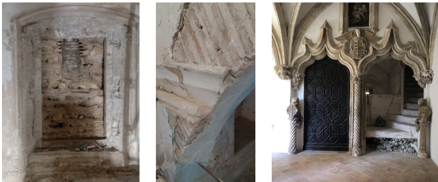
Figure 1. Partitioned façade hole after removing the painting. Springs and carved railings on walls and facade after removing the door, where the overlapped staircase can be appreciated which was later removed to reveal the lower original one. Behind it, the partition on the flamboyant railing. Source: photographs by the author.
