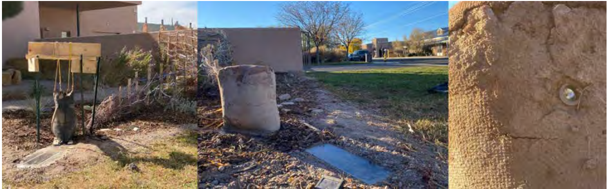
Figure 3: Albuquerque Museum sculptural installation showing formwork, final pour with acrylic covered excavation and detail of surface and detail of agave fiber in mix. (Source: Authors 2021)
