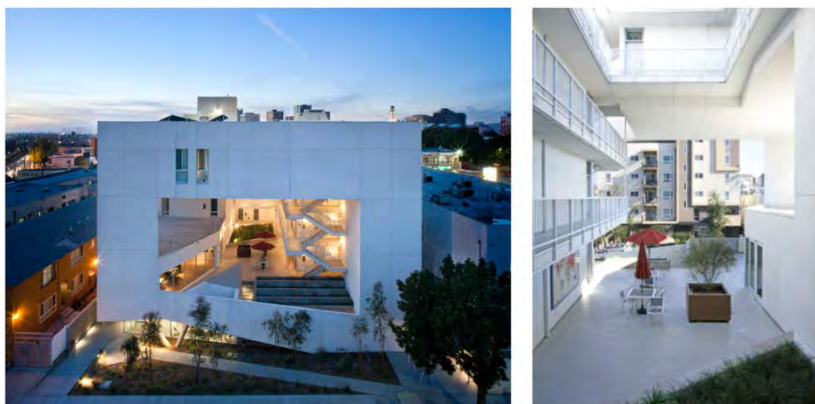
Figure 5: The Six and Courtyard (Photo courtesy of Brooks+Scarpa, source: https://brooksscarpa.com/the-six )
