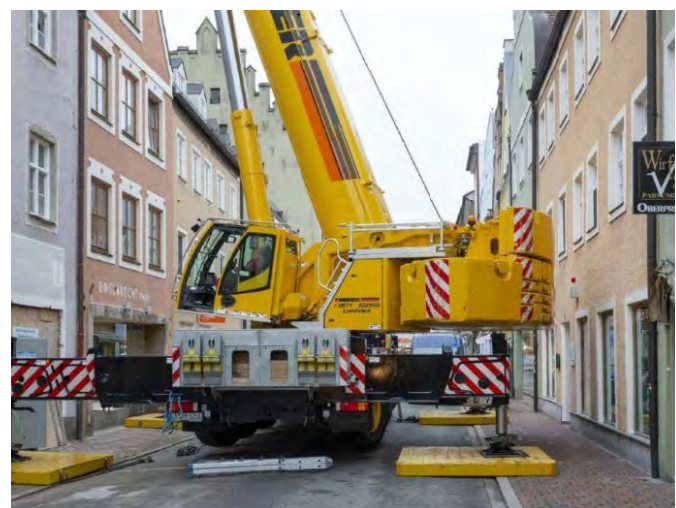
Figure 2: Crane set-up. (Dalhgruen 2012)
