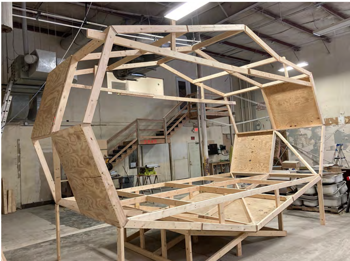
Figure 2: Full-scale construction experiments in light wood framing led to the development of Light Timber Construction.
