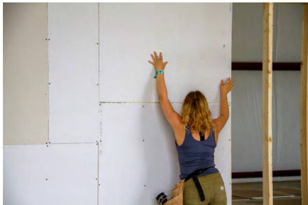
Figure 1: Installation of various gypsum panel sizes. Source: (Author 2020)
