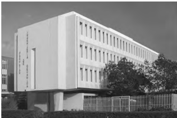
Figure 3. Escuela Politécnica Nacional (EPN), School of Mechanical Engineering, designed by Oswaldo de la Torre. Source: Saltos & Sánchez, 2010.
